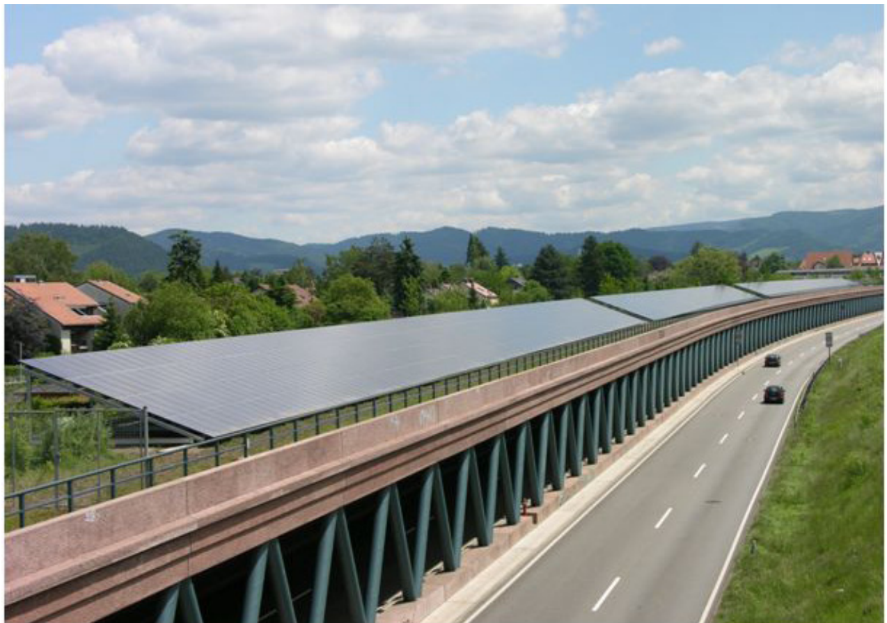
A community-owned PV array on a noise barrier in Freiburg, Germany. Source: fesa GmbH 2006
